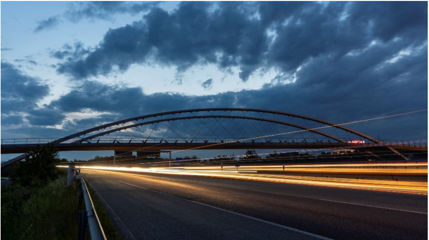
Bridge with CFRP-Hangers (Photo: Andreas Schnubel, sbp)
